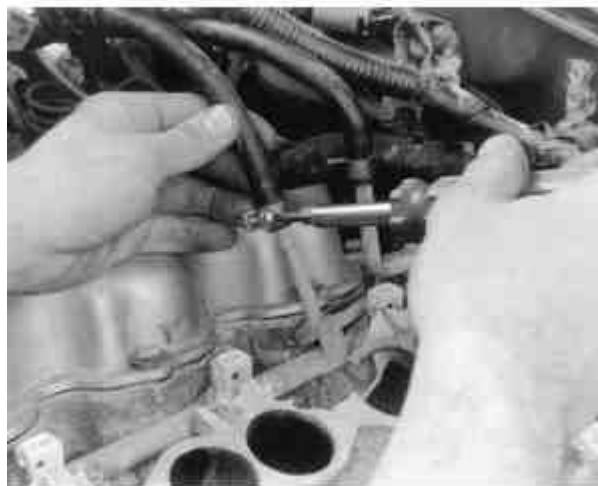
Fig. 13: View of the fuel rail installed — note the location of the pressure regulator assembly
